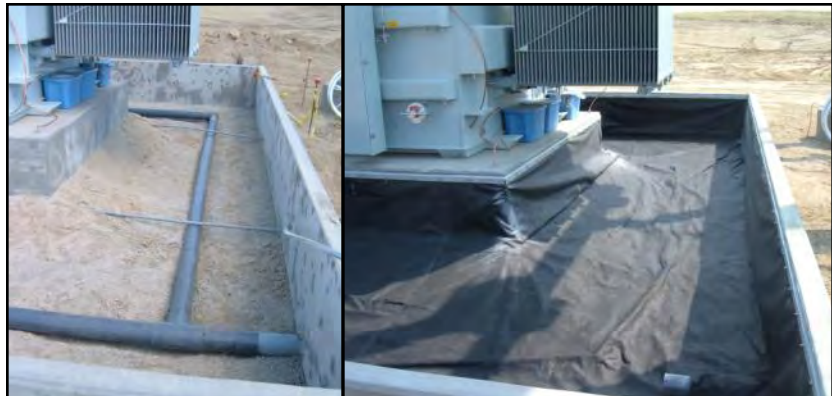
Transformer Pad (Before / After)
