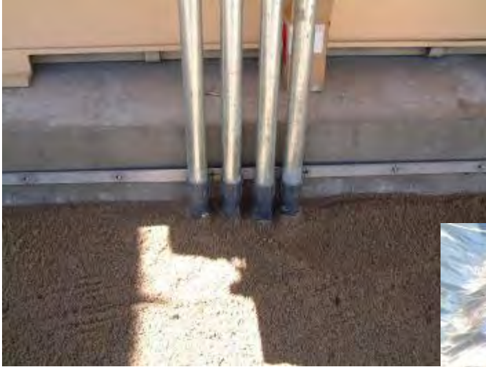
Manifold Boot Before Construction
