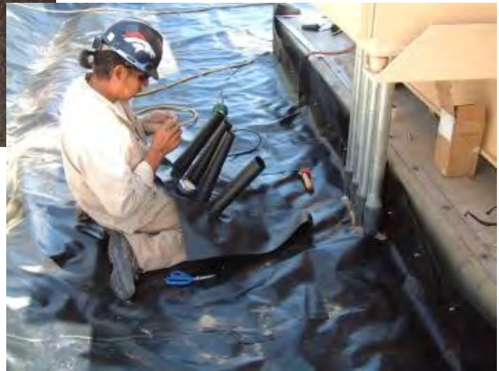
Manifold Boot During Construction
