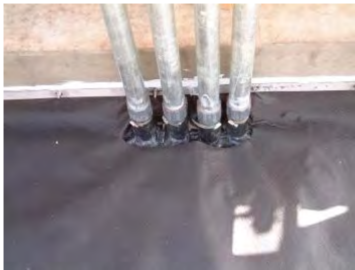
Manifold Boot After Construction
