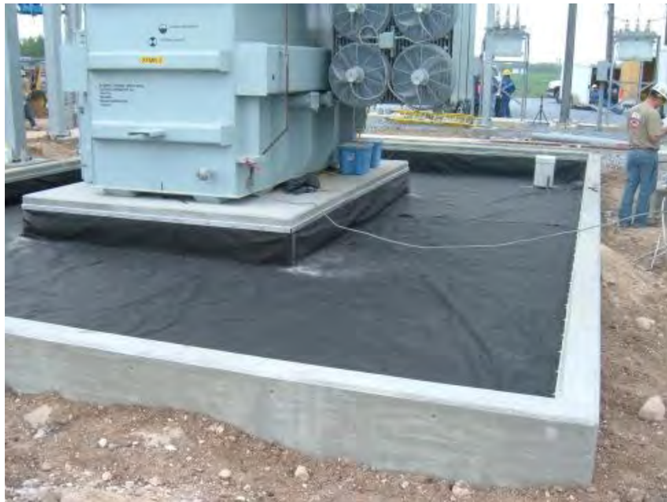
Transformer Pad after to Liner Installation
