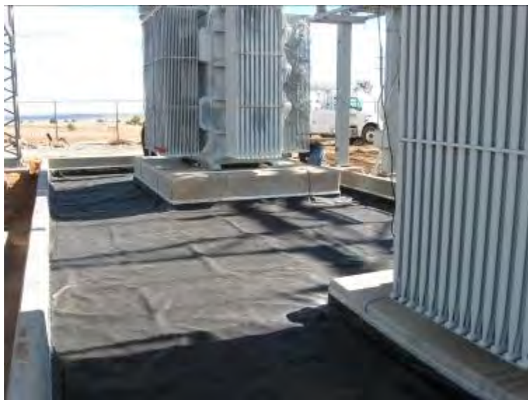
Substation After Liner Installation
