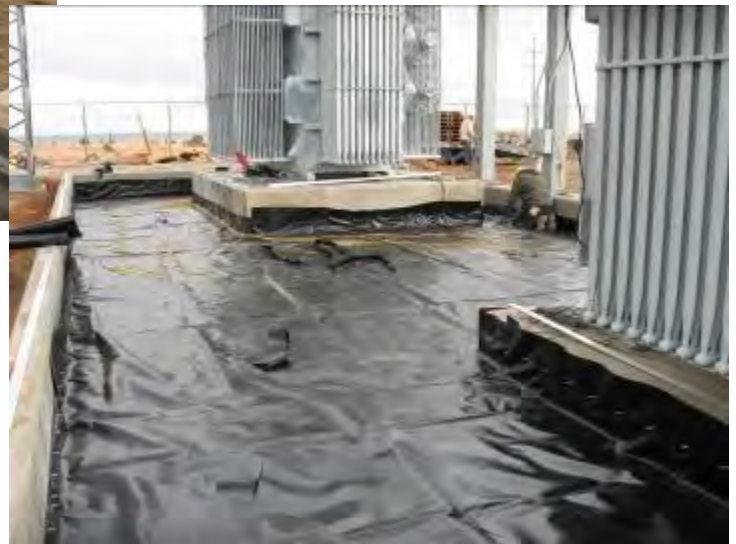
Substation During Liner Installation
