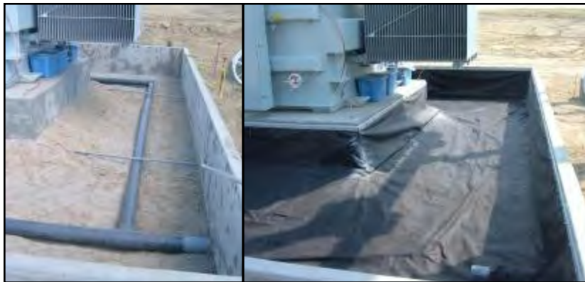
Transformer Pad (Before / After)
