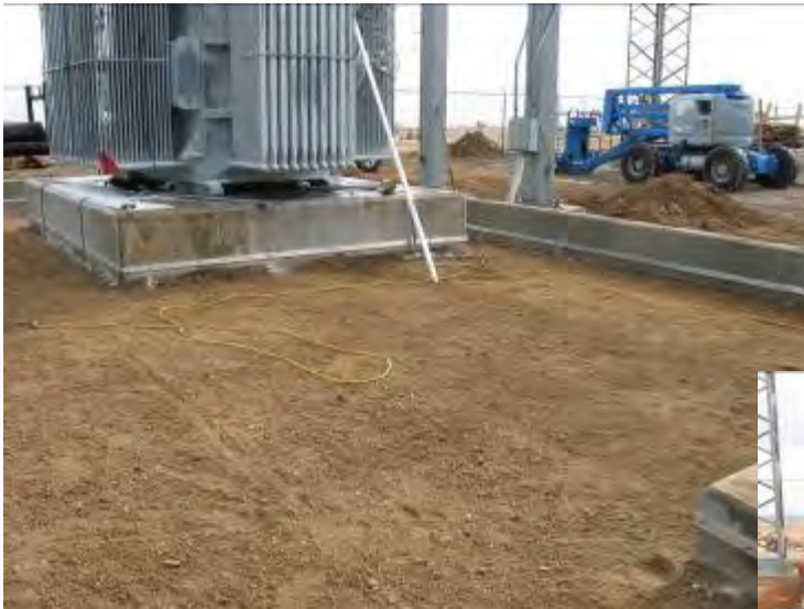
Substation Before Liner Installation
