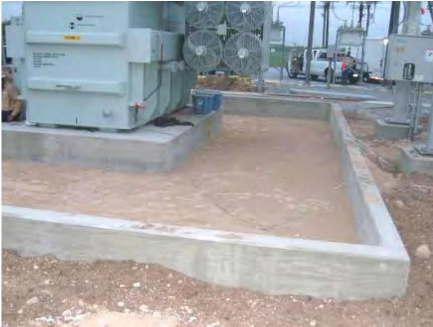
Transformer Pad prior to Liner Installation
